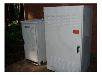
This IdaTech PEM fuel cell system provides back-up power to the Oregon State Police emergency response transmitters. The fuel cell replaces a diesel generator.
