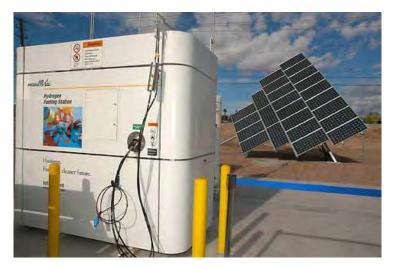
This hydrogen station in Las Vegas, Nevada, uses a solar array to produce hydrogen via electrolysis. The station serves hydrogen vehicles used by the Las Vegas Valley Water Department, and the hydrogen storage is provided by Air Products.
