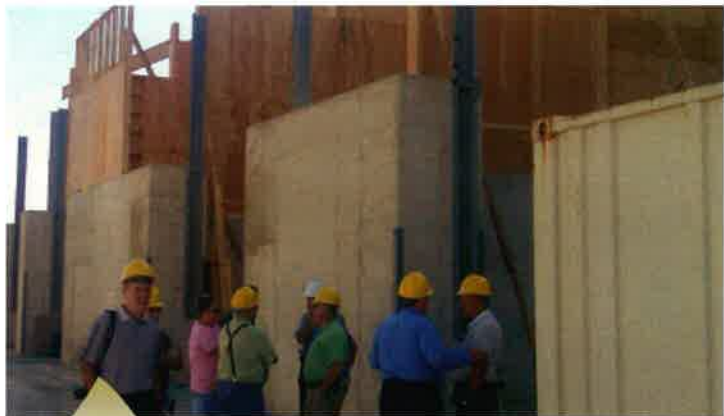
Ag Committee Members Visit the Helena Chemical Construction Site
