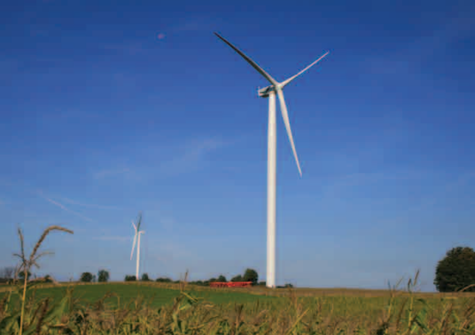
Stoney Corners Wind Farm, McBain, Michigan. Photo courtesy of Jennifer Kempken, Barton Malow Company.
