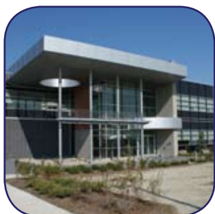
Ajax LEED Fire and Emergency Services Headquarters
